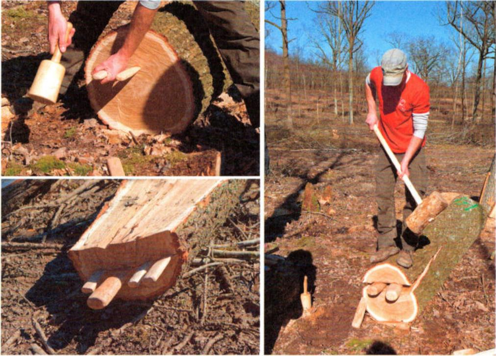
Abb. 7: Tangentiales Spalten (unterschiedliche Versuche). – Splitting tangentially (different trials).
