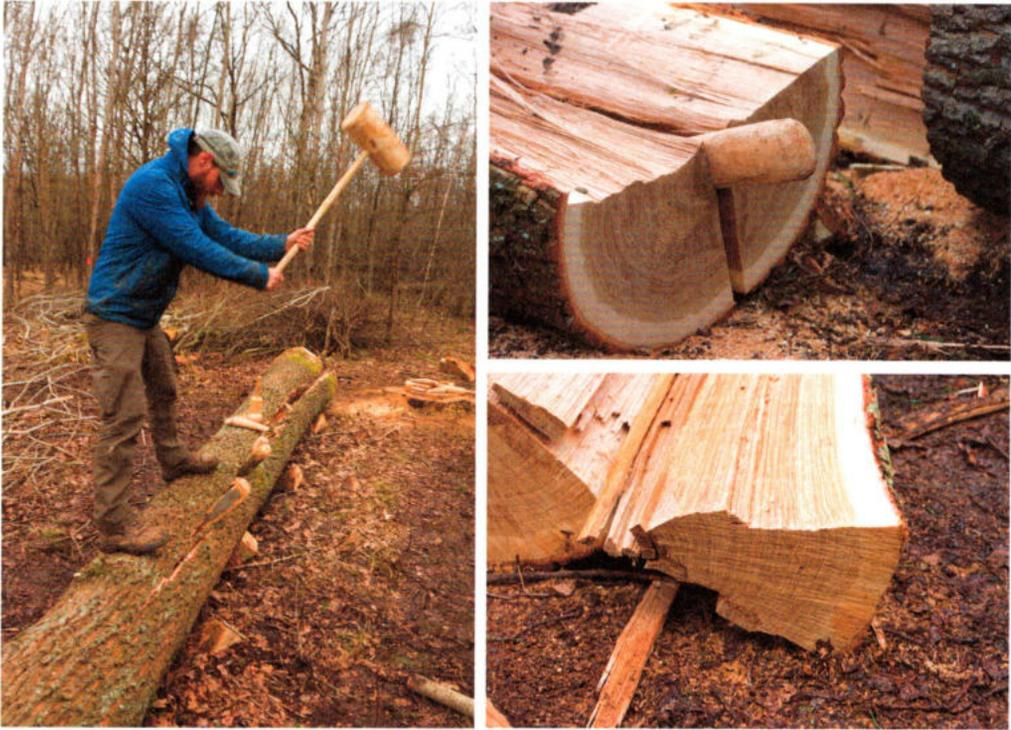
Abb. 5: Radiales Spalten (unterschiedliche Versuche). – Splitting radially (different trials).
