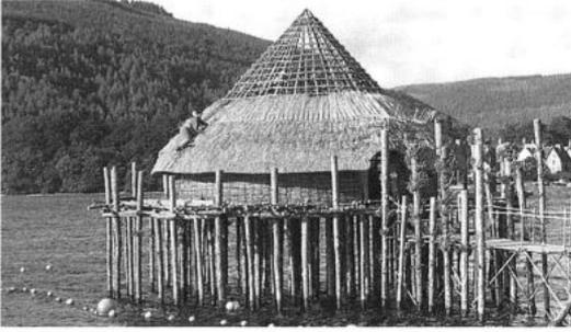
Fig. 17: Thatching the roof.
