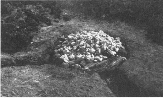
*Fig. 4: A lime burning kiln at Lemba in the process of firing. The kiln is 1.0 m in diameter.*
