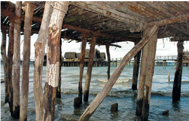
▼ Fig. 27: Supporting pile under the Horn- staad recons- truction in the Pfahlbaumuseum Unteruhldingen.
