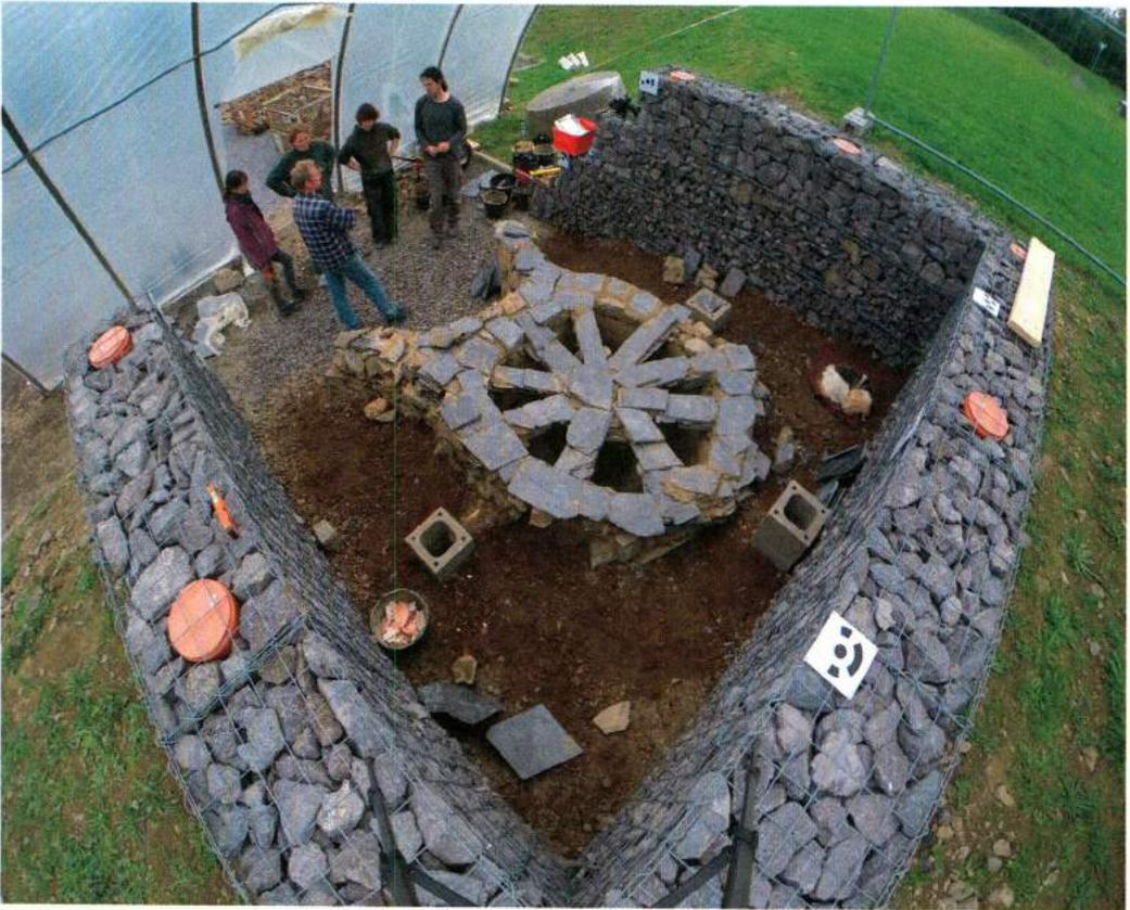
Fig. 5: Construction of the perforated floor using overlapping slabs of slate. – Bau der Speichertenne aus überlappenden Schieferplatten.
